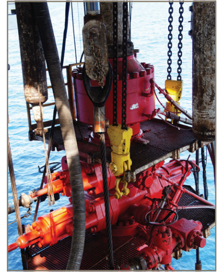
BOP - safety critical and operationally dependent upon clean fluids
